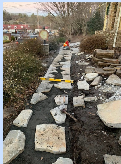
A flagstone path being installed in the Norcross Garden Club Cottage Garden.
