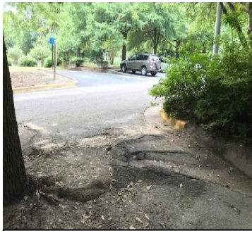
Broken Pavement at the entrance to the Azalea Walk in October 2020
