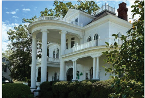
Magnolia District HLP 2026, Tour of Historic Dublin
